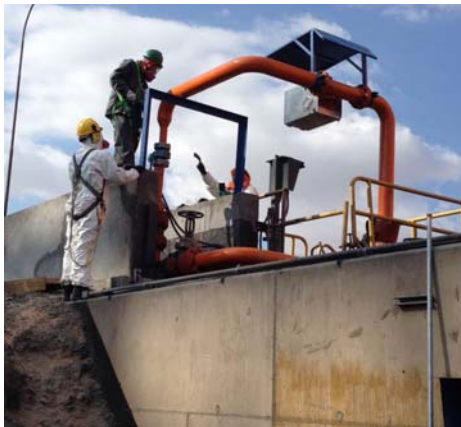
Figure 1. MV-21-N Direct on line mounting
